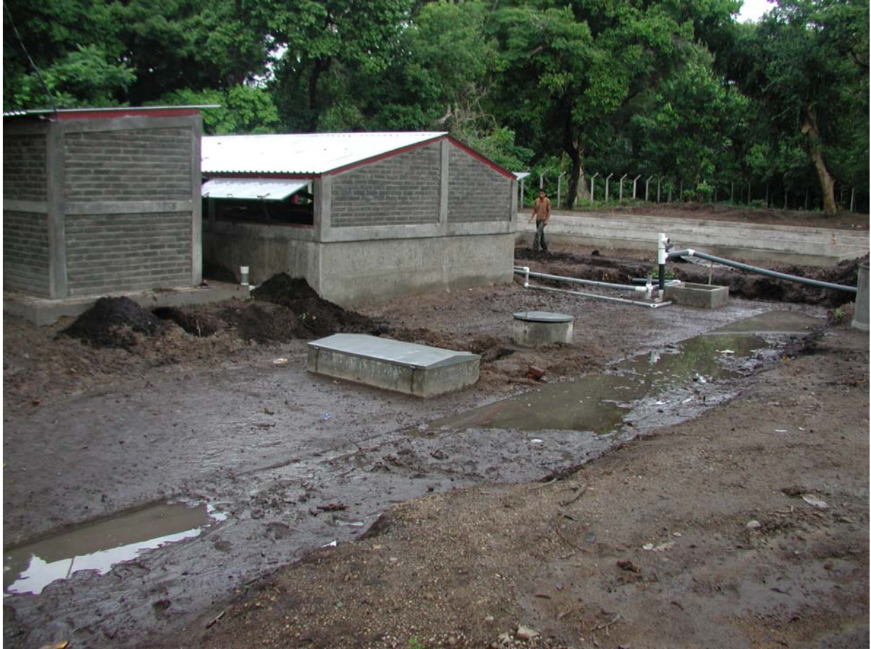
Treatment Center, Approaching Completion
