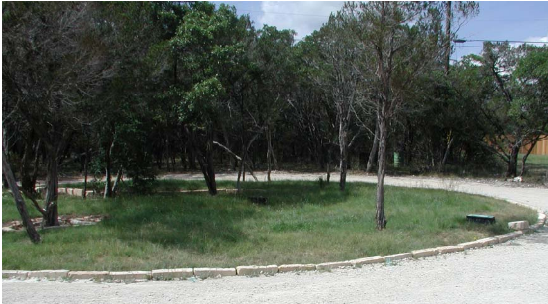
Driveway Island Area of Drip Field, During and After Installation
