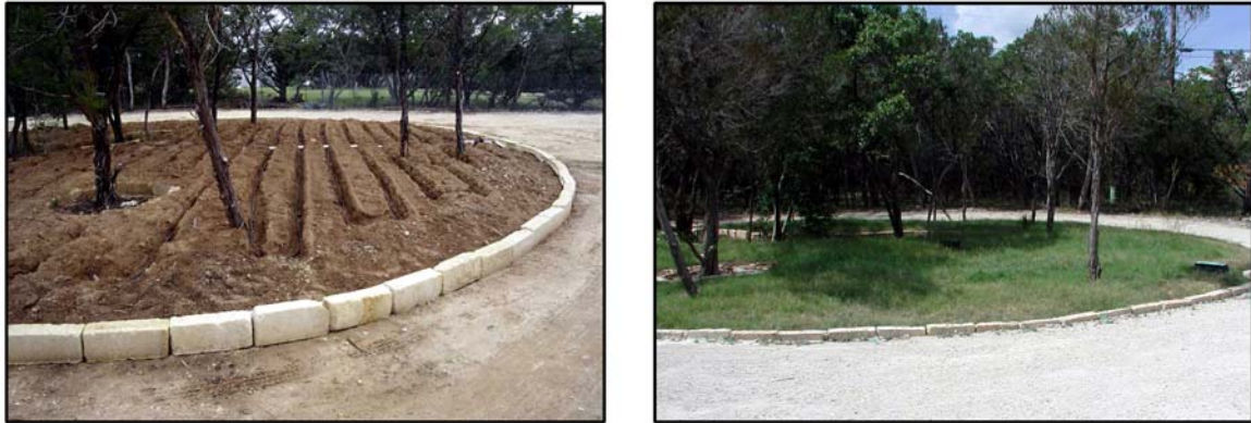
Fig. 7. SDI Field During Installation and After Completion
