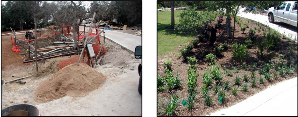
Fig. 9. Field Area Before and After Installation and Landscaping
