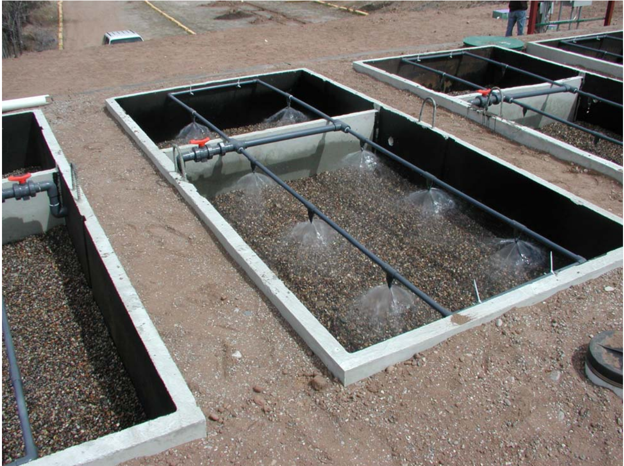
Filter Bed with Media Installed, Spray System Being Tested
