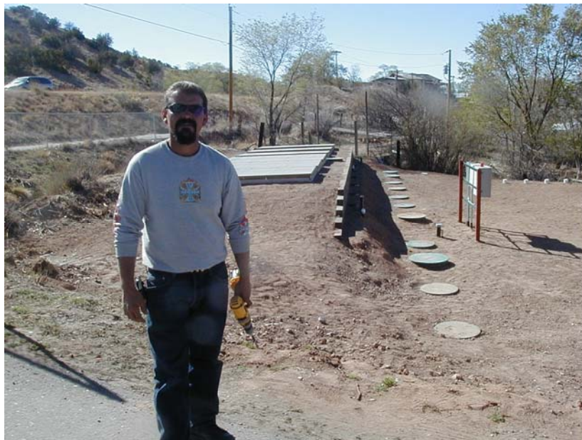
The Treatment Center Showing the Filter Bed Covers
